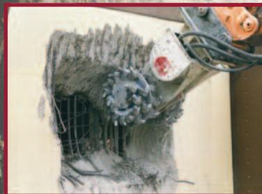
AQ-5 Demolition Project AQ cutting attachments can cut up to one inch rebar
