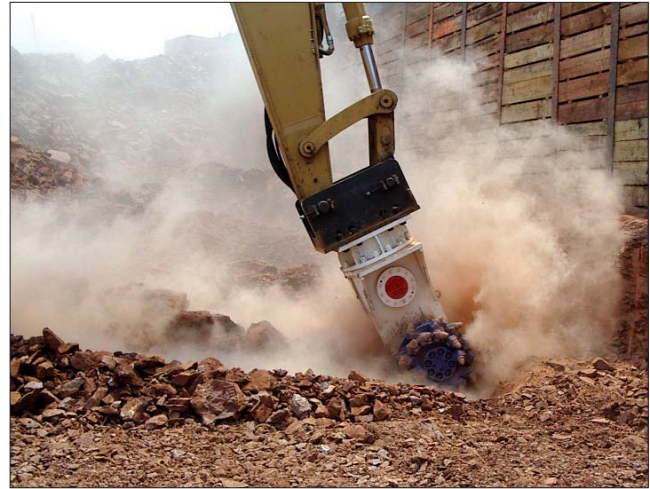
Specialized hydraulic rock grinding/cutting attachments (pictured) have become increasingly popular for exact scaling and profiling, but still fall short of the mass production that can be achieved by roadheaders.
